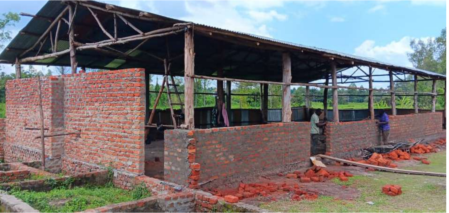
Church building under construction
